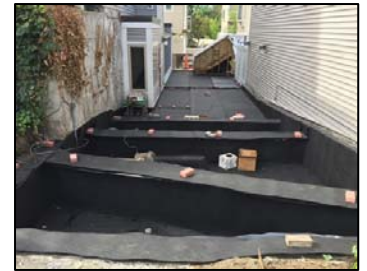
The concrete slab was assumed to be a stepped slab, but was actually a flat slab with concrete beams of varying height supporting the treads
