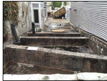
The concrete slab was assumed to be a stepped slab, but was actually a flat slab with concrete beams of varying height supporting the treads
