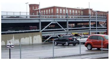
To maintain safe, uninterrupted access for residents, the team completed the lower two levels by working a half-level at a time, using fencing and signage to safely and efficiently reroute traffic.
