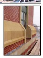
**THE PROCESS:** The building was first staged with full-height pipe staging, and netted for life safety measures and to protect the surrounding area. Many of the precast concrete elements around the tower had begun to fall and in some cases fallen to the ground.
