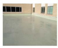
**Photo 1:** An appropriate surface primer was applied, and the new fluid-applied system was hand applied to the concrete deck, with a blown-glass in-mat form incorporated into the system to provide crack bridging and durability.
